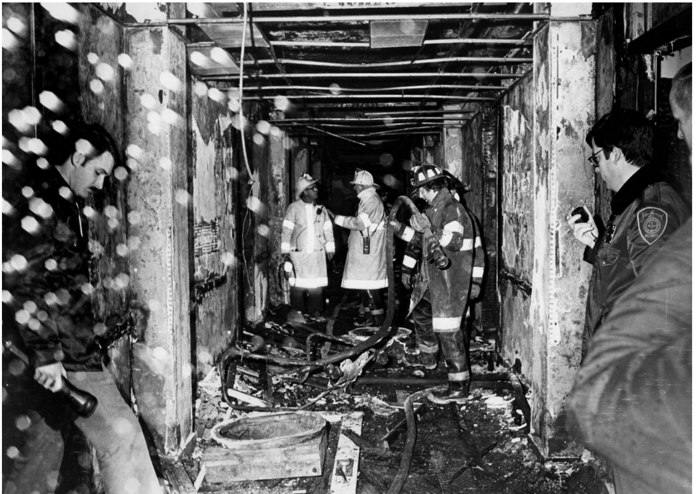
The third floor of the Copley Plaza Hotel where the fire started. WILLIAM BRETT/GLOBE STAFF/FILE
